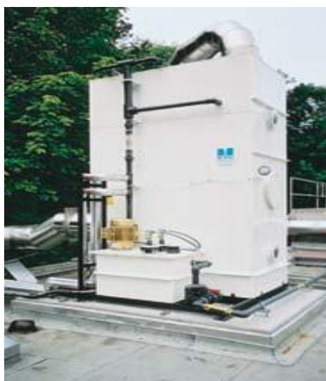
Figure 7 Packed Bed Scrubber
