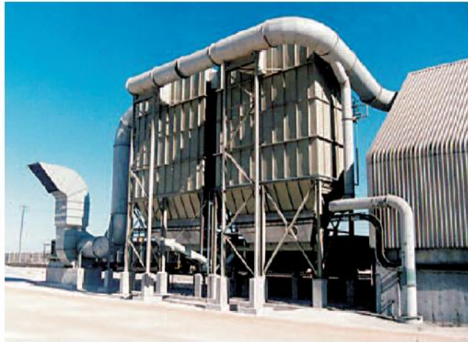
Figure 1: Reverse Air Bag Filter
