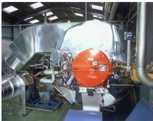
Figure 11: Thermal Oxidiser
