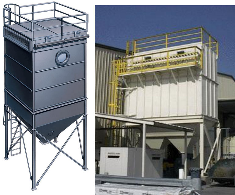
Figure 2: Pulse-Jet Bag Filter
