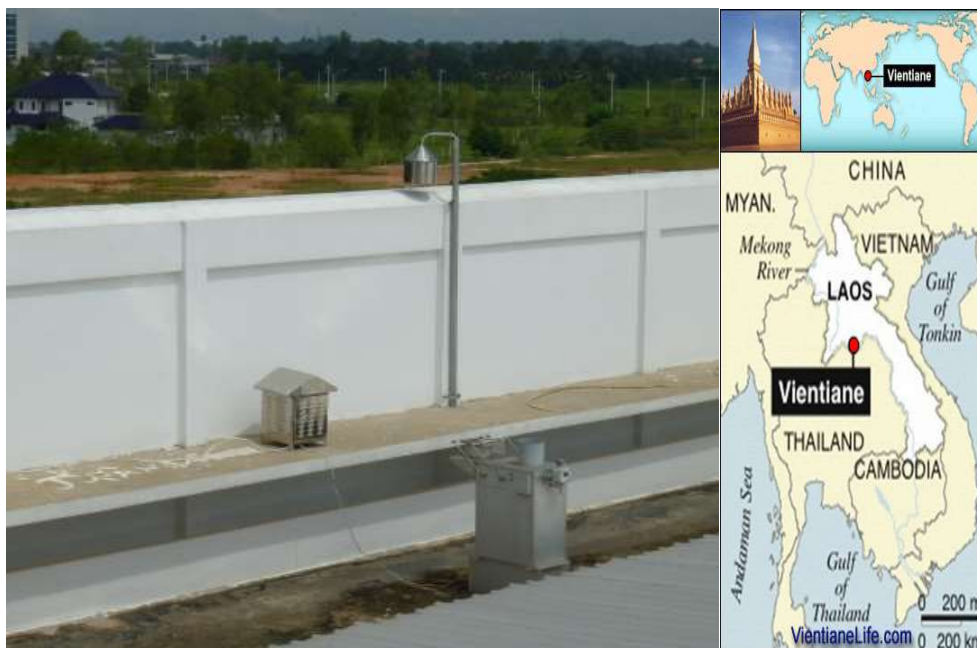
Figure 1.1. Monitoring station for wet and dry deposition.
